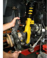
23. Install the lower strut bolt finger tight.
